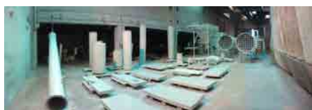
Sabbatura e verniciatura Sandblasting and painting of components
